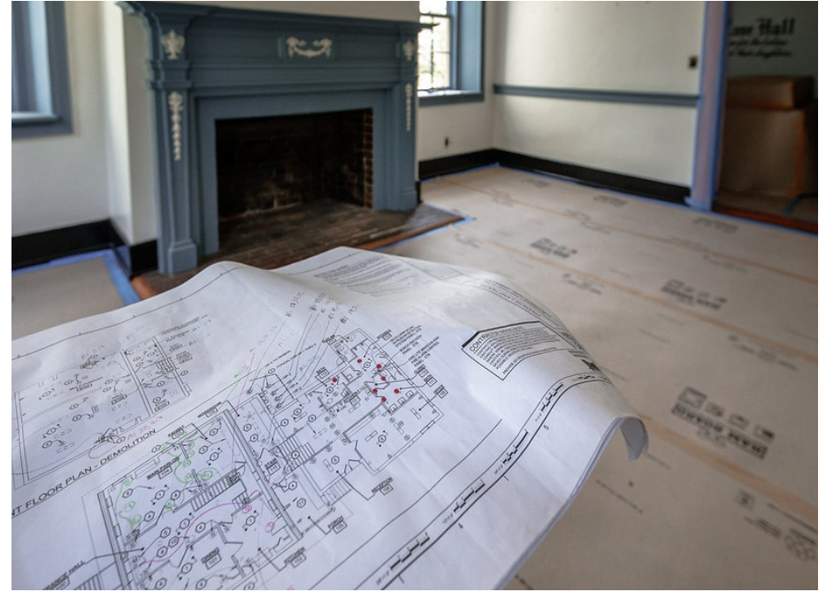
Restoration Work at Francis Land House
